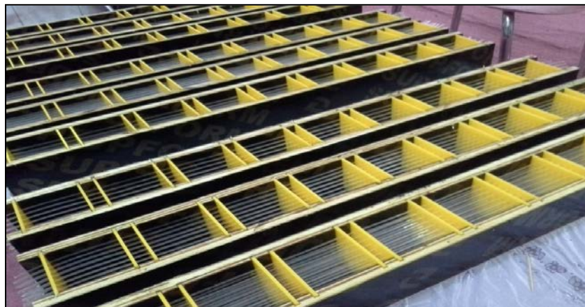
Figure (4): Details of cubes of wood mold after fixing the POFs.
