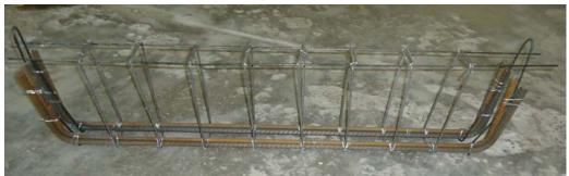
Figure (3) Steel reinforcement cage used for beams construction
