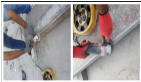
Figure 6: Smoothing the concrete corners prior to fix CFRP strips
