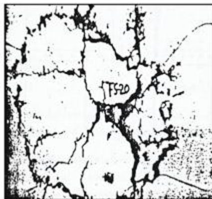
Figure 9: Experimental crack pattern of slab FS-20 [6]
