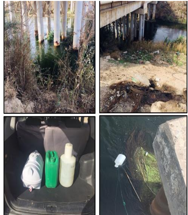
Figure 4: water source in general drain water and the filled up tanks
