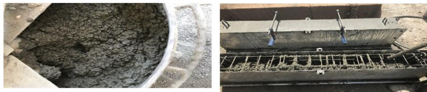
Plate 1: Mixing procedure of concrete and casting of the beams
