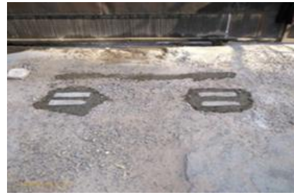
Fixing process of sensors into the holes Figure 5: Continued
