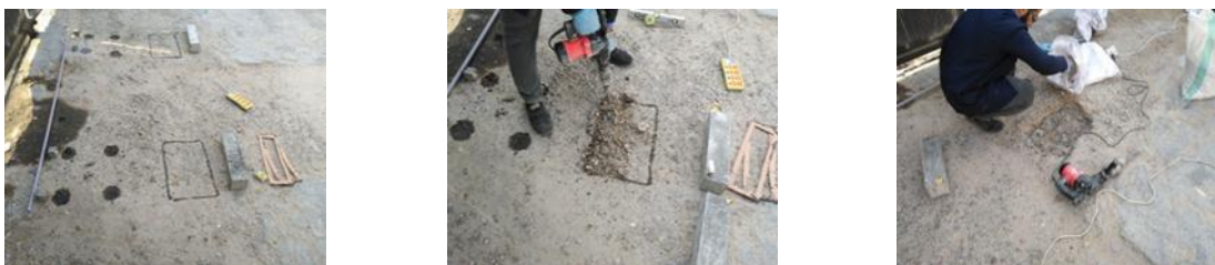
Marking and excavation process
