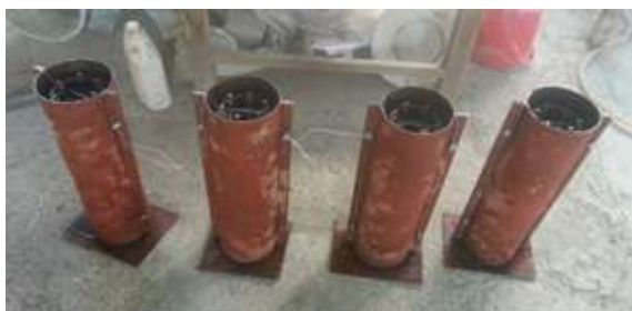
Figure 2: Assembled column moulds
