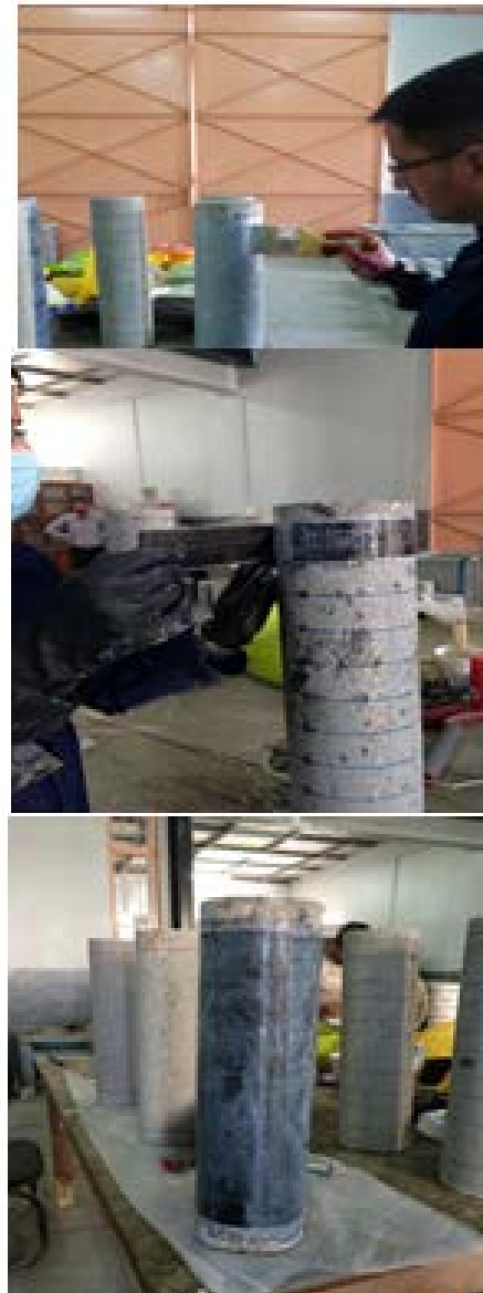
Figure 4: Application of CFRP
