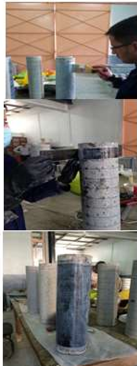
Figure 4: Application of CFRP
