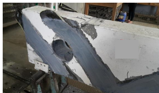
Plate 6: Failure mode and tearing of CFRP strip for B4-R-I
