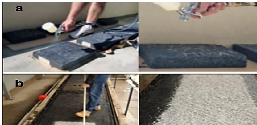
Figure 4: (a) The \text{TiO}_2 solution spraying process (b) the painting process of \text{TiO}_2 solution [43]
