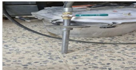
Plate 4: The tube for cement grouting
