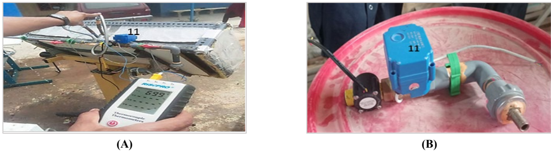
Figure 3: A- shows the connection of the E.C.S (11) on the water pipe joining the faucet and its effect on the temperature of water discharged from the solar collector, which was measured with a thermocouple device. B- The electronic control system is connected to the cool water pipe
