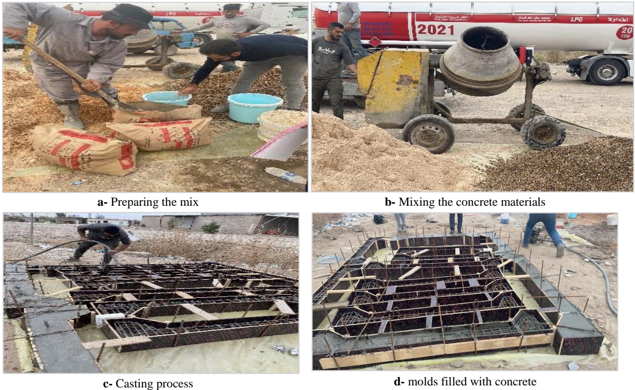
Figure 4: Concrete mixing and casting process, a- Preparing the materials quantity to mixing the concrete to cast test columns, b- Concrete mixing process ,c- Tested columns casting in wood forms, d- Tested columns after casting
