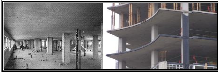
Figure (1) Flat Plate Constructions (Nilson, 2004)
