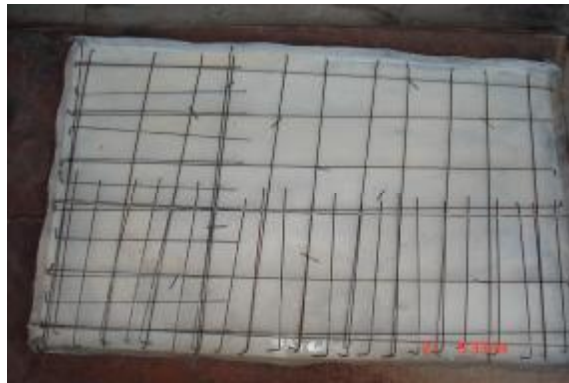
Photo (4) Details of the reinforcement mesh of slab S_4 (case 4).
