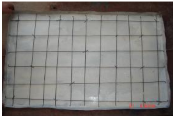
Photo (2) Details of the reinforcement mesh of slab S_1 (case1).
