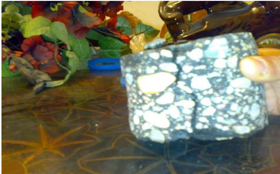
Plate (1) Field Core Extracted From Asphalt Concrete Pavement
