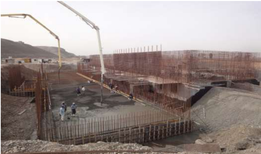
Figure (1) Low Lift Pump station (Pump House under construction).
