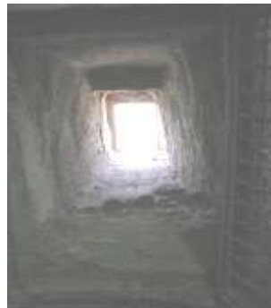
Figure (9) Small opening (window) through the thick wall providing ventilation and light.
