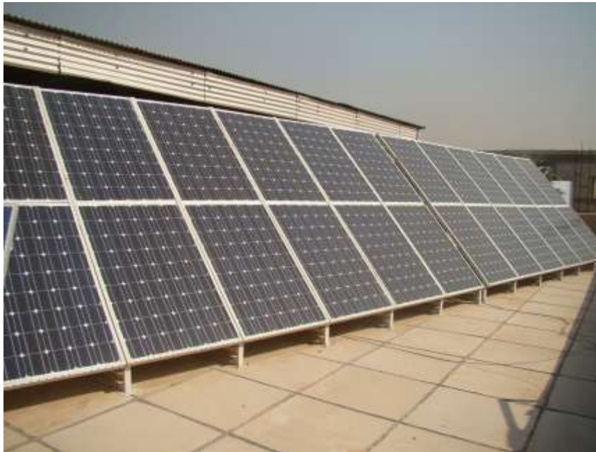
Figure (1) installation of 24-monocrystalline silicon PV modules.
