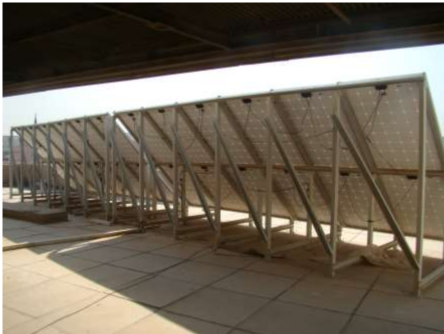
Figure (4b) positioning array tilt angle ( \alpha ) in relation to the horizontal plane.
