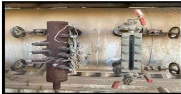
**Figure 5:** The gauge of the water level in the (Al-Quds power plant).
